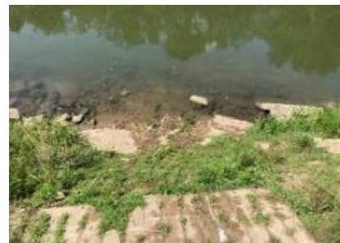
Ramp washout at Retz Wildlife Area Access
